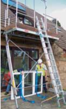
Attaching the new window
