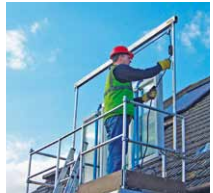
Hoisting to final position
