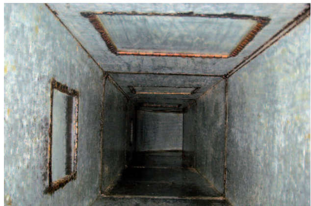
Kitchen extract duct after cleaning
