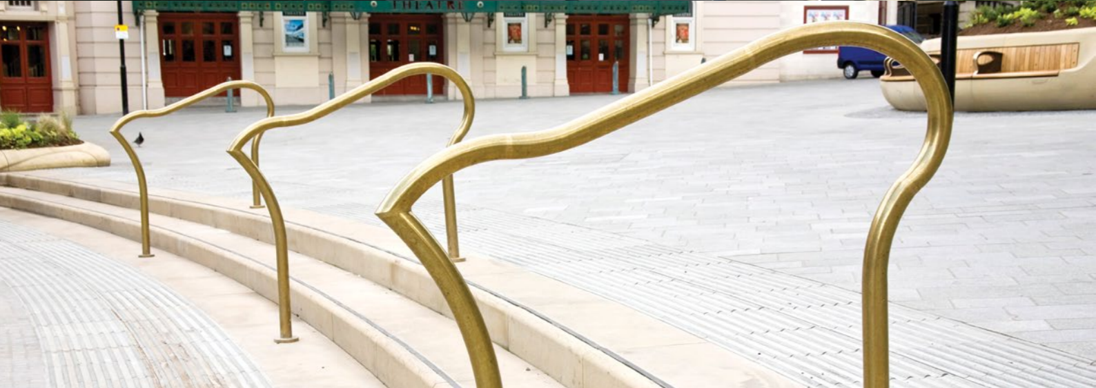
RAMP AND BALUSTRADE TO FOOTBRIDGE – M20 JUNCTION 9
