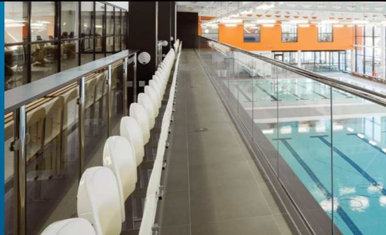
STRUCTURAL GLAZED BALUSTRADE TO SEATING AREA
