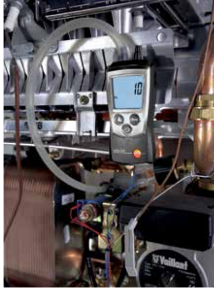
Fig. 9: Reading the gas connection and nozzle pressure on the testo 510
