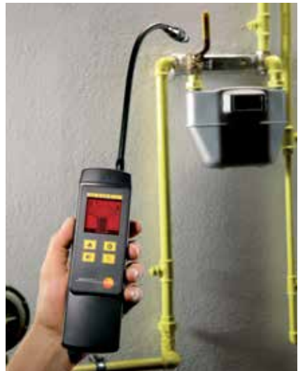
Fig. 20: Leak detection on gas pipes using the testo 316-2
