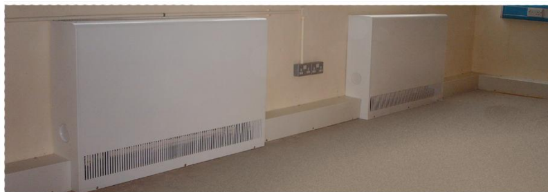
Refurbishment Project - After
