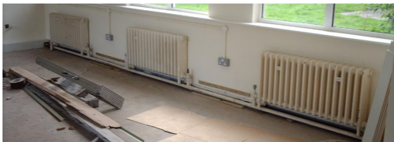
Refurbishment Project – Before
