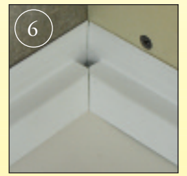
6 Check notches and corner joints meet
