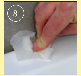
8 Clean ledge using Sealux alcohol wipes
