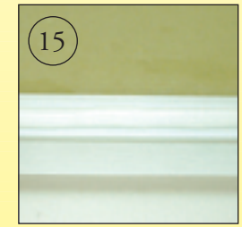
15 Lay Sealux-N bead across strip upstand
