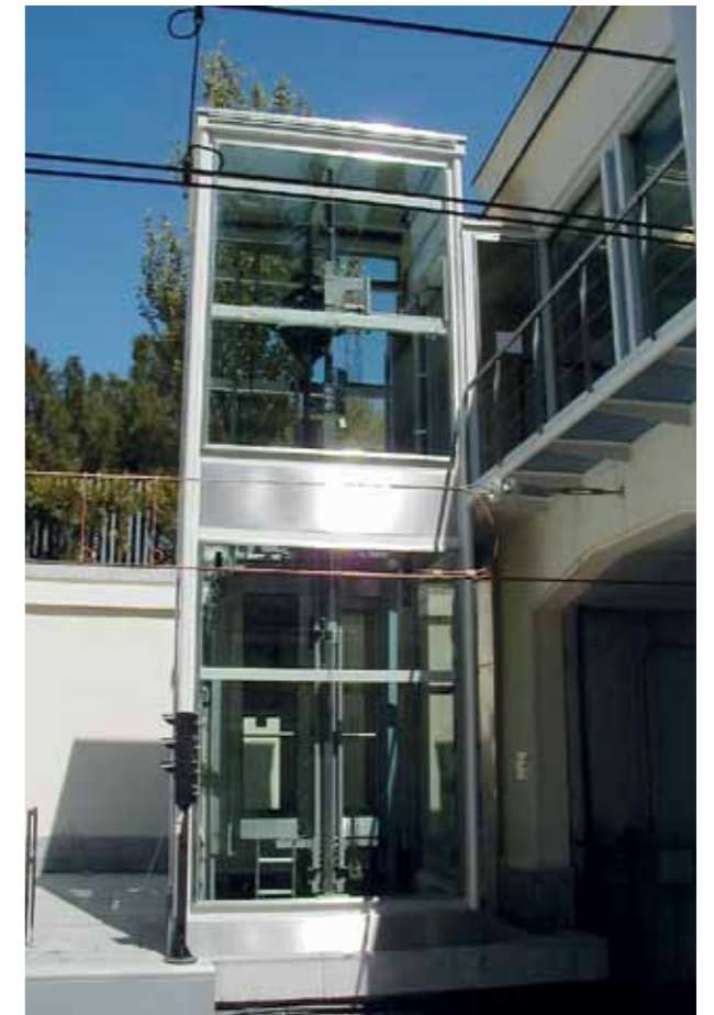
Figure 3. Self-standing steel shaft
