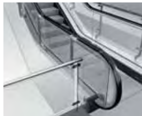
Passenger fall protection barrier height up to 1300 mm.
