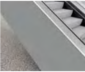
Grey primed sheet steel cladding (RAL7036) *
