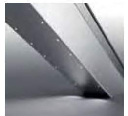
Soffit spot lighting
