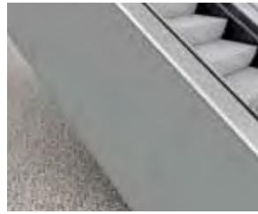
Grey powder coated sheet steel cladding (RAL7036) ***
