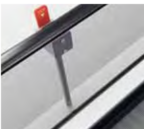
Additional emergency stop button (EN115-1:2008:+A1:2010 requirement)
