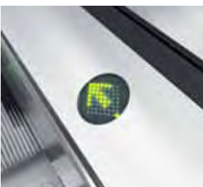
LED traffic lights located in the decking
