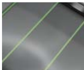
Pallet demarcation lighting
