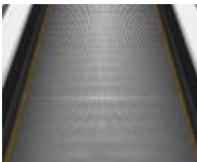
Yellow painted demarcation on two sides of pallet
