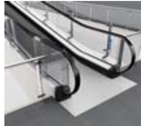
Passenger fall protection barrier height up to 1300 mm. Recommended when a fall greater than 6 m is possible
