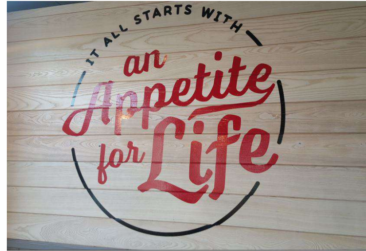
Specialist 3M 8624 heat activated self adhesive film applied to faux brickwork and timber feature walls.
