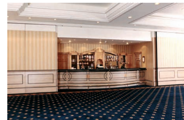
Monoplan Type 100 S finished with skirting, panelling, dado, and wall covering.
