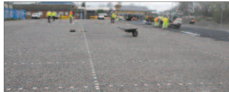
Completed parking area
