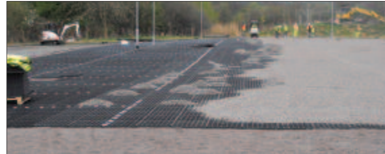
Parking area under construction
