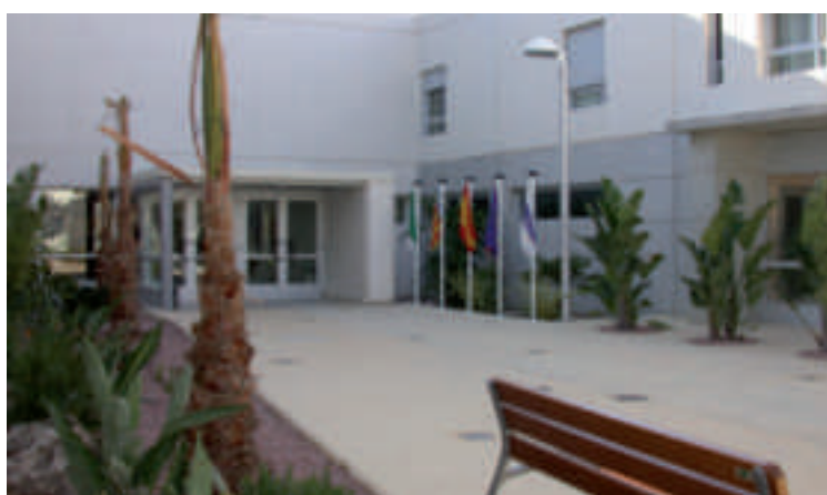
Vincente del Raspeig retirement home, Valencia, Spain
