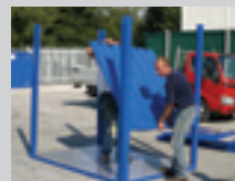
4. INSERT THE SIDE WALL PANELS
