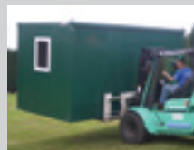
2. ASSEMBLED UNIT CAN BE TRANSPORTED BY TRUCK OR FORKLIFT, OR LIFTED FROM ITS LIFTING EYES BY CRANE
