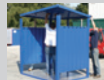
6. LIFT ON AND FIX THE ROOF
