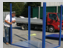
3. FIT CORNER POSTS TO THE BASE
