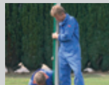
3. FIT THE FOUR CORNER POSTS
