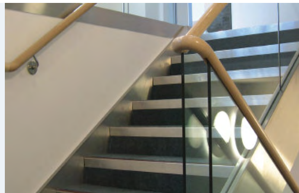
Crystal balustrade and Natura handrail with satin polished stainless steel trim
