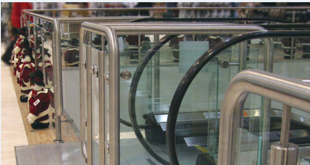
Stainless steel Onyx balustrade and toughened glass infill panels
