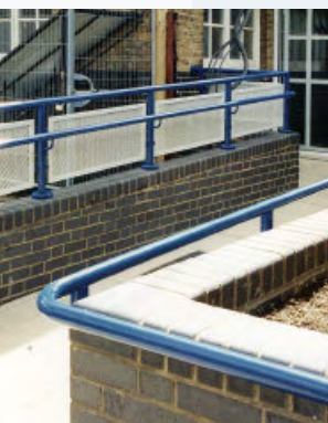
Coral balustrade with perforated panels to a ramp
