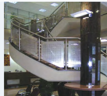
Onyx balustrade on helical staircase with curved, satin polished stainless steel perforated panels
