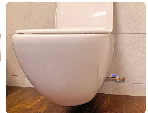
* PipeSense sends data to the portal via the Irus room ControlSensor using Bluetooth.
