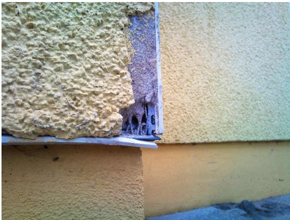
Images 3 & 4: Steel beads are prone to damage from external sources which can leave unpleasant, and in some cases dangerous, damage to render integrity.
