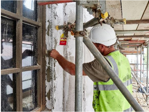
Images 1 & 2: Renderplas PVC beads offer builders a better, safer and stronger alternative to traditional steel beads.
